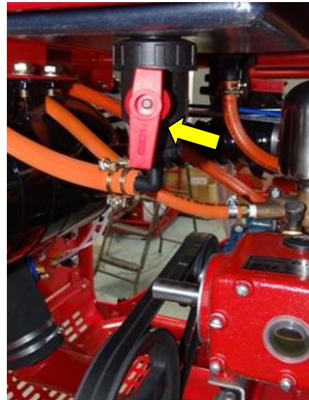
Before opening the filter, shut the formulation line ball valve (shown here in open position).
